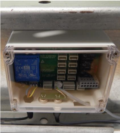
Vertical mounting, in this case well protected by the journal of the yoke
